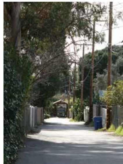
Alleys provide opportunities for the installation of powerlines and other utilities, keeping them away from the fronts of neighborhood streets.
