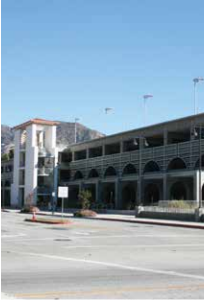
Los Angeles Mission College converted their surface parking lot into a multiple story parking structure as part of their Master Plan.
