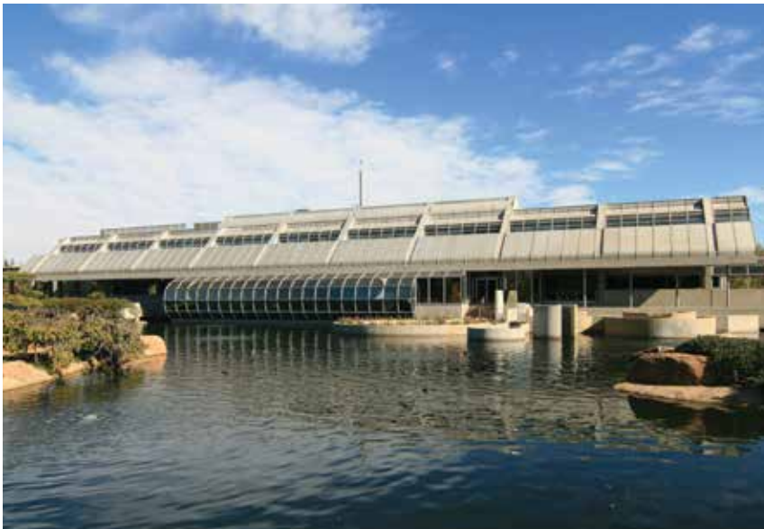
The Donald C. Tillman Water Reclamation Plant processes approximately 80 million gallons of waste per day as it purifies wastewater and produces recycled water. Photo Credit: You-are-here.com
