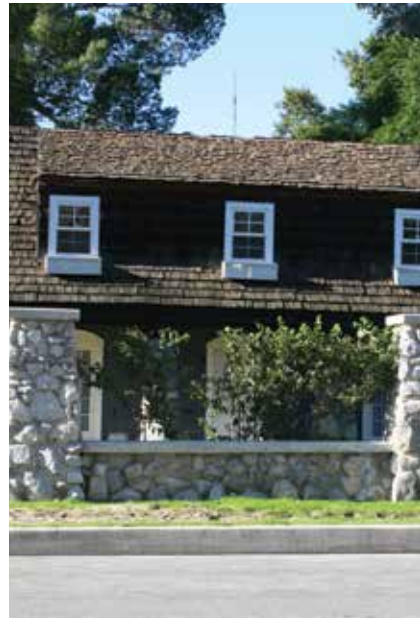
Sylmar contains a number of homes that reflect the historic character and architecture of the Sylmar community.
