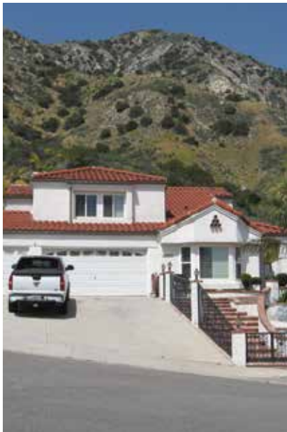
Constructing single-family homes below significant mountain ridgelines will preserve the scenic views of the hillsides in Sylmar.
