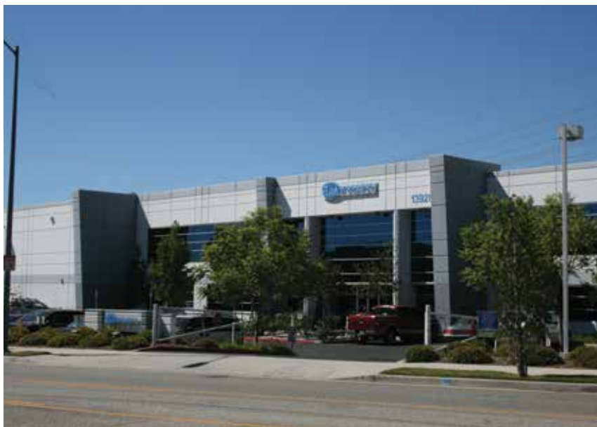
Encourage and support environmentally friendly businesses within the industrial areas of the community.
