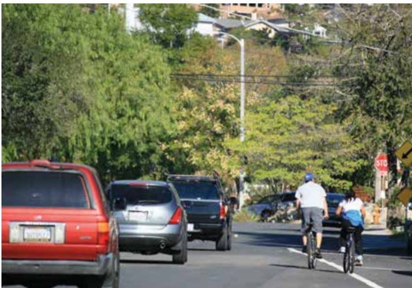
Wide outside travel lanes provide adequate on-street space for bicycles and vehicles to share the lane without requiring the vehicle to leave its lane to pass the bicycle.
