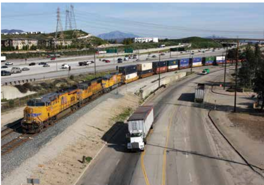
Southeast view from Balboa Bridge overlooking San Fernando Road, the rail-road tracks, and the I-5 and 210 freeway interchange, one the nation's busiest corridor. Photo Credit: Charles Freericks
