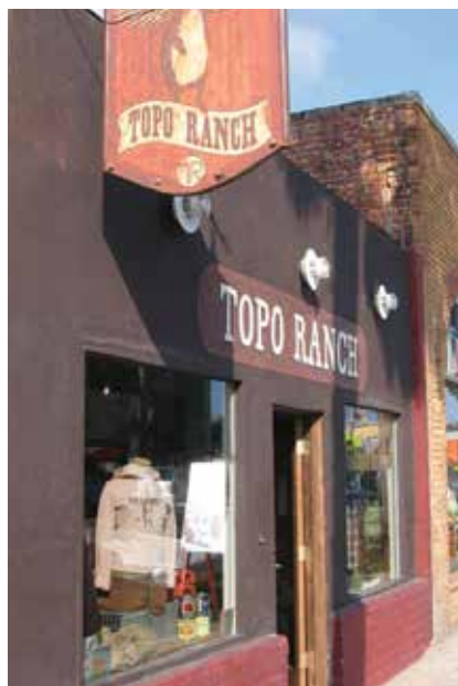
Commercial development incorporating the use of earth tone colors and natural materials helps reinforce the community's character.
