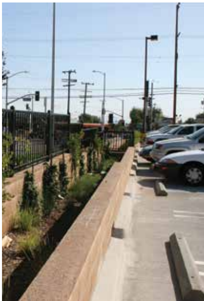
The visual impact of a commercial parking areas can be reduced by providing a buffer like a planter box with landscaping.
