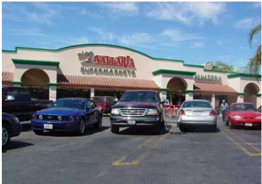
Spanish-style architecture is a common feature in Sylmar’s commercial centers.
