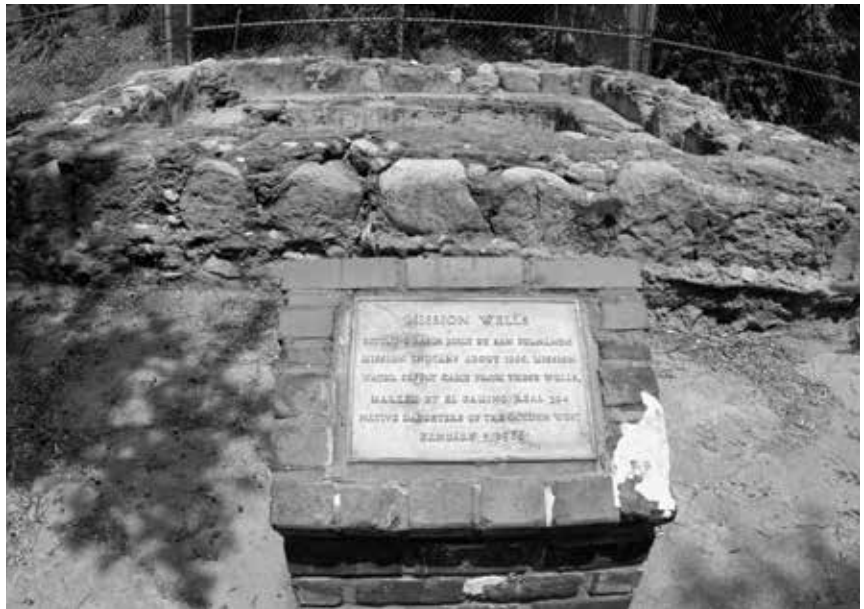
Mission Wells and Settling Basin, Los Angeles Historic-Cultural Monument No. 50.
