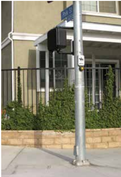
When trails intersect roads, safety is the most important factor. Installing a second push button signal actuator allows users to control the traffic light and safely cross the road.
