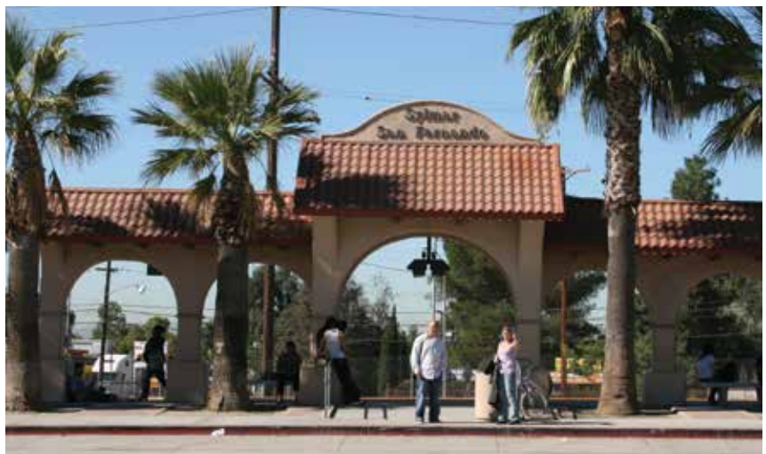
The Metrolink Station located in Sylmar serves as a multi-modal transit terminal and transfer point for bus riders.
