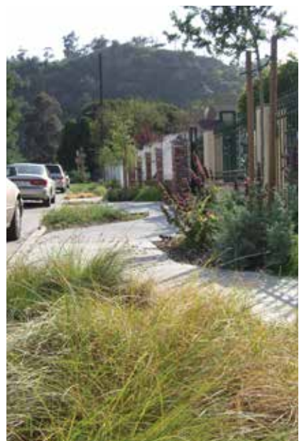
Bioswales in the streetscape design of a neighborhood can increase storm water infiltration and remove pollution and silt from surface runoff water.
