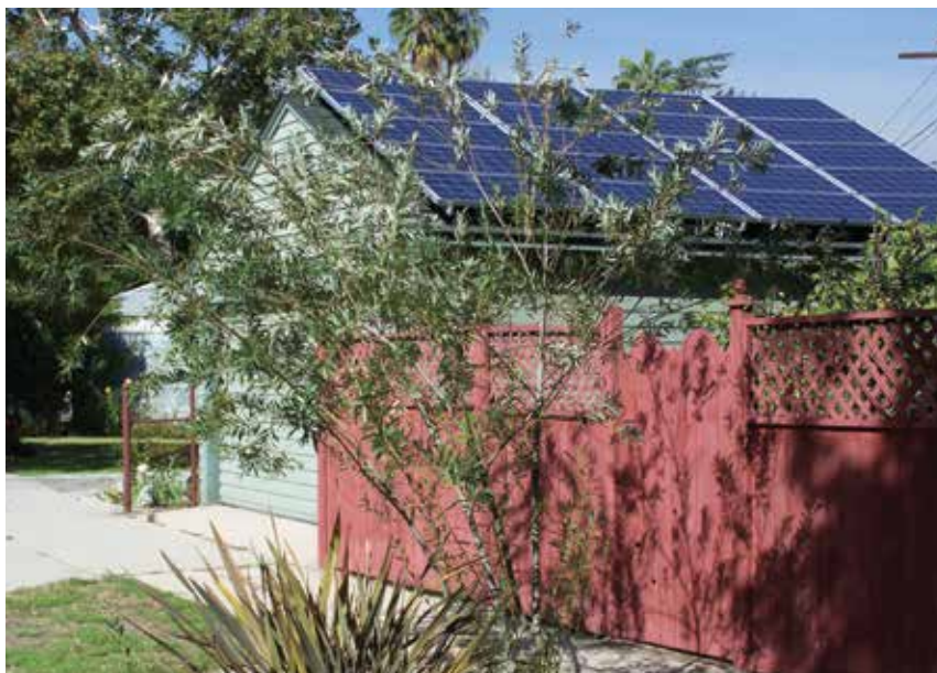
Residential solar panels promote environmentally-friendly power, using renewable energy from the sun. Solar panels can add value to a project when integrated appropriately.
