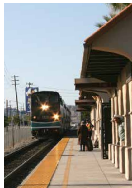
Sylmar's Metrolink Station serves as a multi-modal transit terminal and transfer point for users of public transit.
